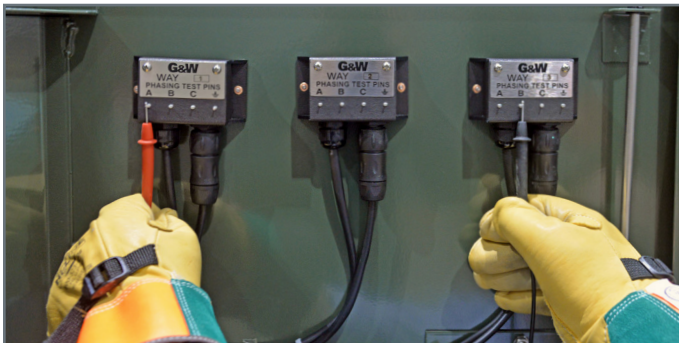
▲ Example of phasing confirmation test performed.
