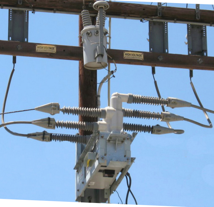
Pictured from top to bottom: Substation mount, standard center-pole mount, alley-arm with Z modules
