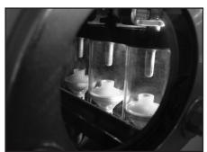
▲ Load break switch visible break.
