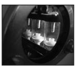
■ Load break switch visible break.
