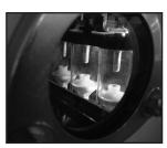
■ Load break switch visible break.
