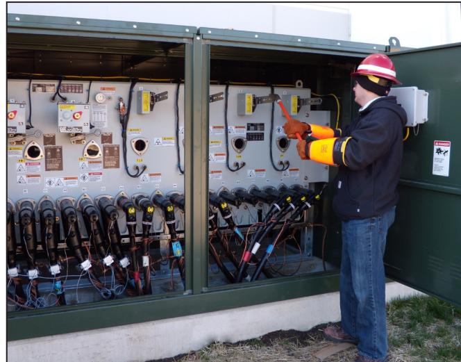
Figure 3: G&W PNI style switch with two automated source ways, three load ways and an additional way for PT protection only.
