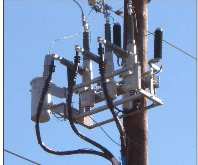
Figure 1: Viper-ST recloser with SEL-651R controls were installed on the two overhead lines.
