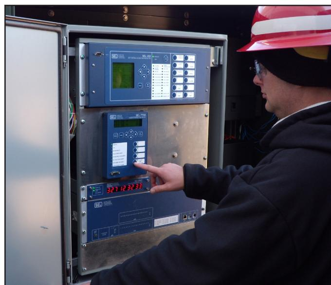
Figure 4: SEL RTAC master was mounted in the same enclosure as the SEL-451 control.
