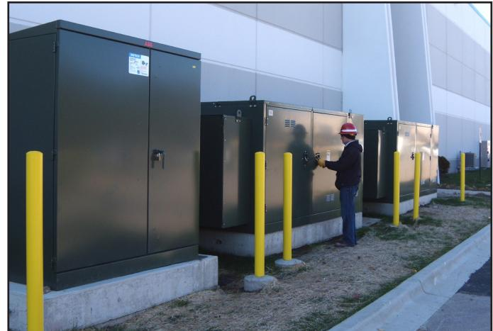
Figure 2: G&W padmount switches and transformers were installed on opposite sides of the building.
