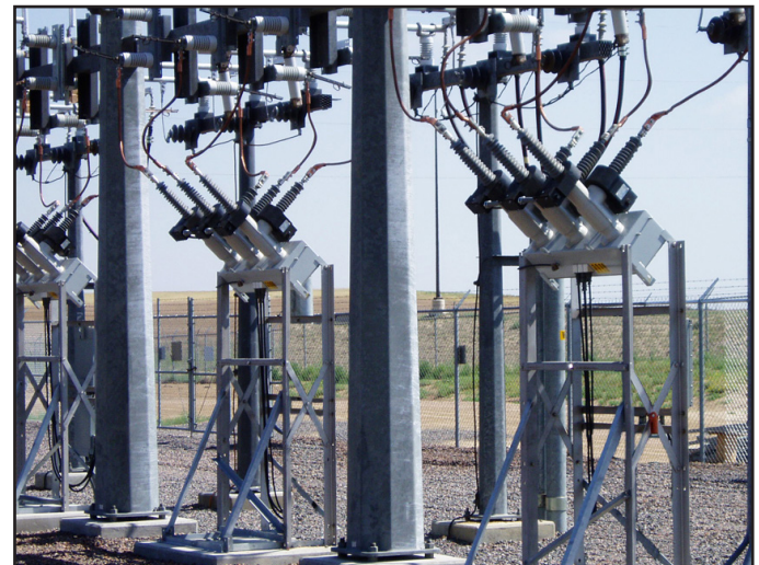
Viper-S reclosers installed in utility substation.
