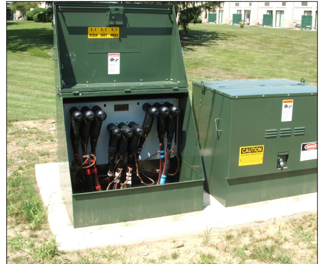
The compact cabinets incorporated a flip-up, padlockable cover for easy access to elbow connections..
