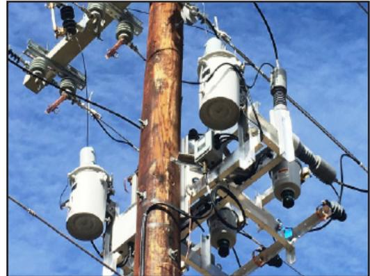
Viper-ST recloser with 6 VS, two control power PTs, and SEL-651R control
