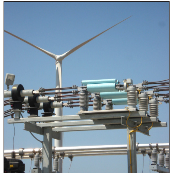
38kV current limiting protectors mounted at the utility grid substation protects the utility from potential wind farm faults and the wind farm from potential utility faults.
