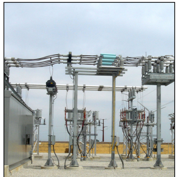
38kV current limiting protectors mounted at the utility grid substation protects the utility from potential wind farm faults and the wind farm from potential utility faults.
