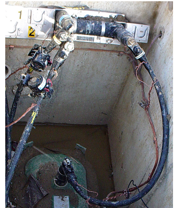
Typical installation showing a 3-position feed-through application in a submersible vault.
