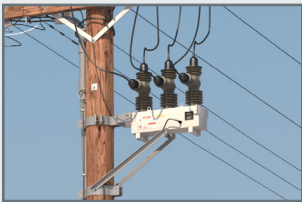
Three Phase Overhead Load Break Switches
