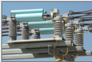
System Protection Equipment
